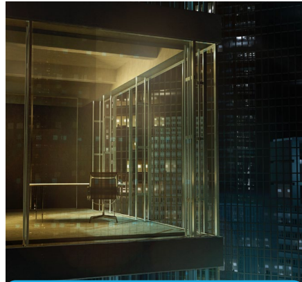
Energy Management, Maintenance, Security
